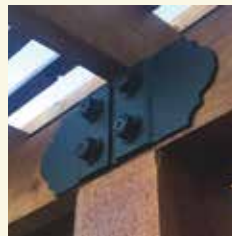
Butt Joint Flush
