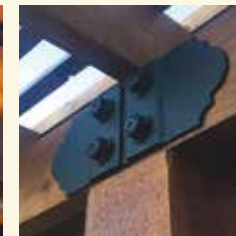
Butt Joint Flush
