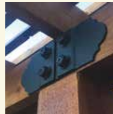
Butt Joint Flush
